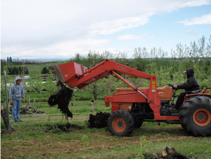
Ripping stumps out with a backhoe at Tukey Orchard, Pullman, WA (June, 2009).
