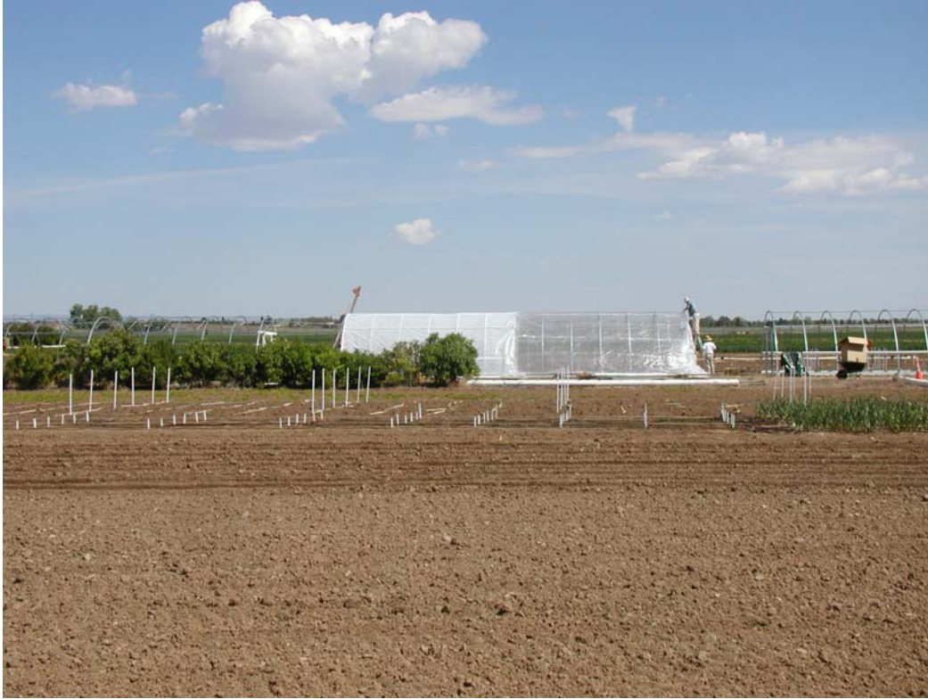
Construction of OFRF screened tunnel project. CSU 5/2006.
