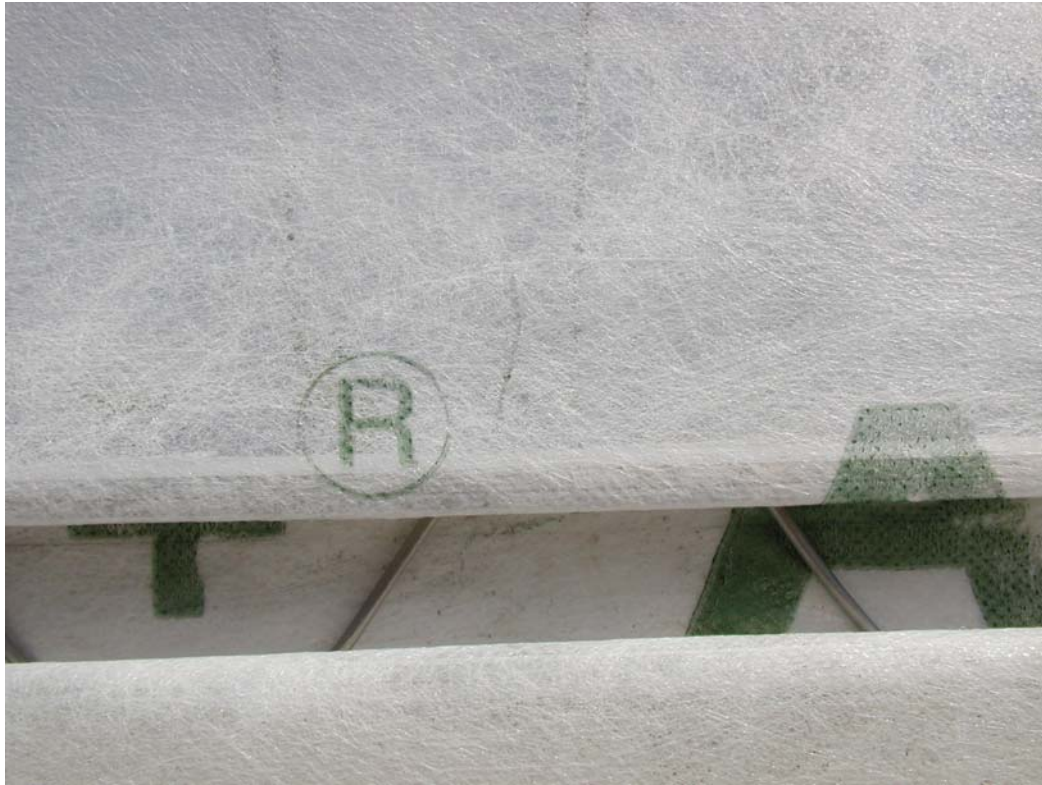
Wiggle-wire holding SBP to frame of high tunnels. CSU 5/2006.
